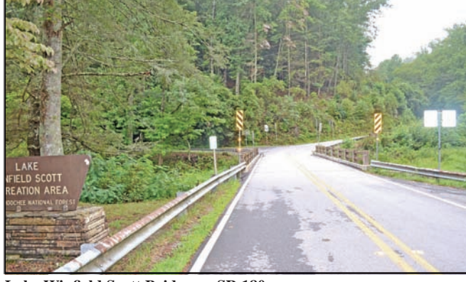
Lake Winfield Scott Bridge on SR 180
